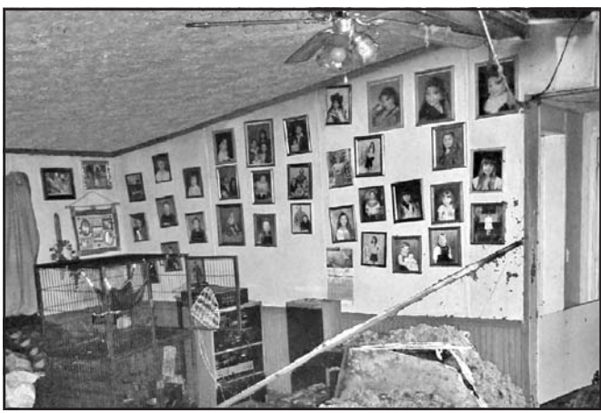
The fire department was able to save the family photos and belongings of this home on King Cove Road.
